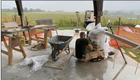
The staff finished renovation of the Knight Prairie Pavilion which included replacement of the wooden support posts with steel beams and then building limestone columns around the beams. Dave Gustafson, **Assistant Operations** Superintendent, did most of the stone work which required significant custom detail for mounting the interpretive panels.
